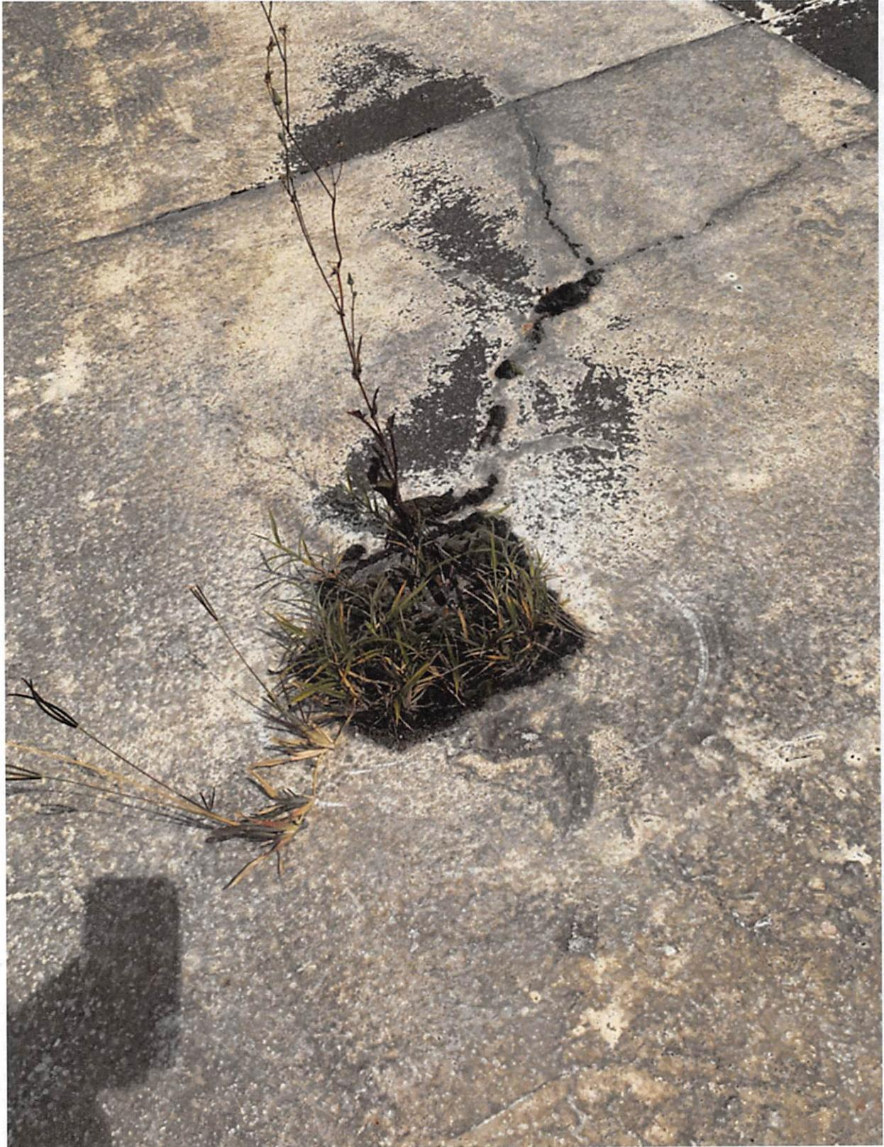
PMB HELOPAD ROOF DRAIN BLOCKED WITH GROWTH
