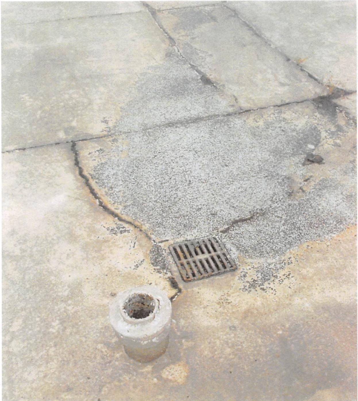
PMB HELOPAD ROOF/SURFACE IS CRACKING
