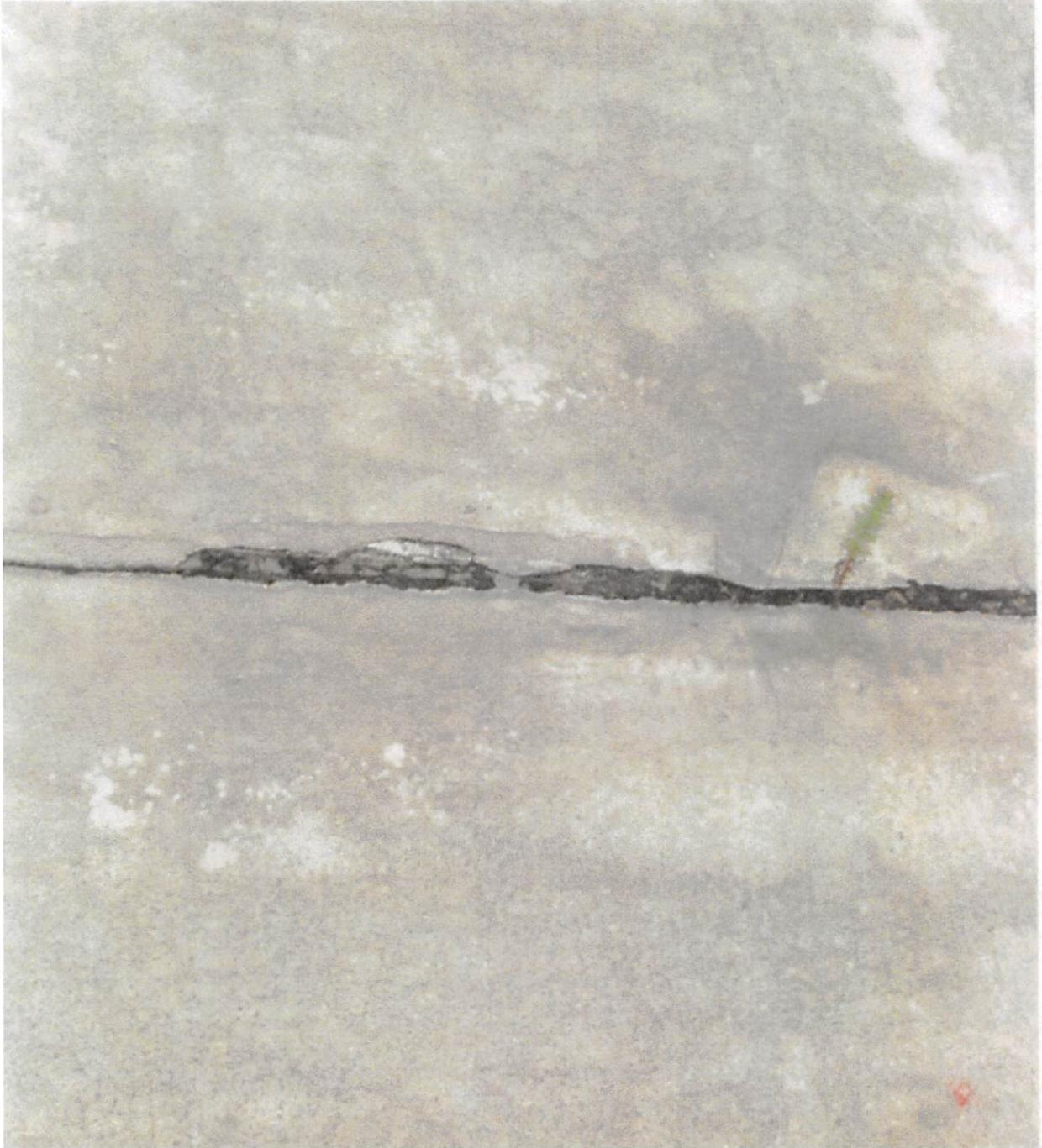
PMB HELOPAD ROOF/SURFACE IS CRACKING AND WEEDS ARE GROWING. LARGE PIECES OF ROOF FLAKING OFF. POSSIBLE HAZARD FOR HELICOPTER OR PERSONNEL DURING TAKEOFF AND LANDING
