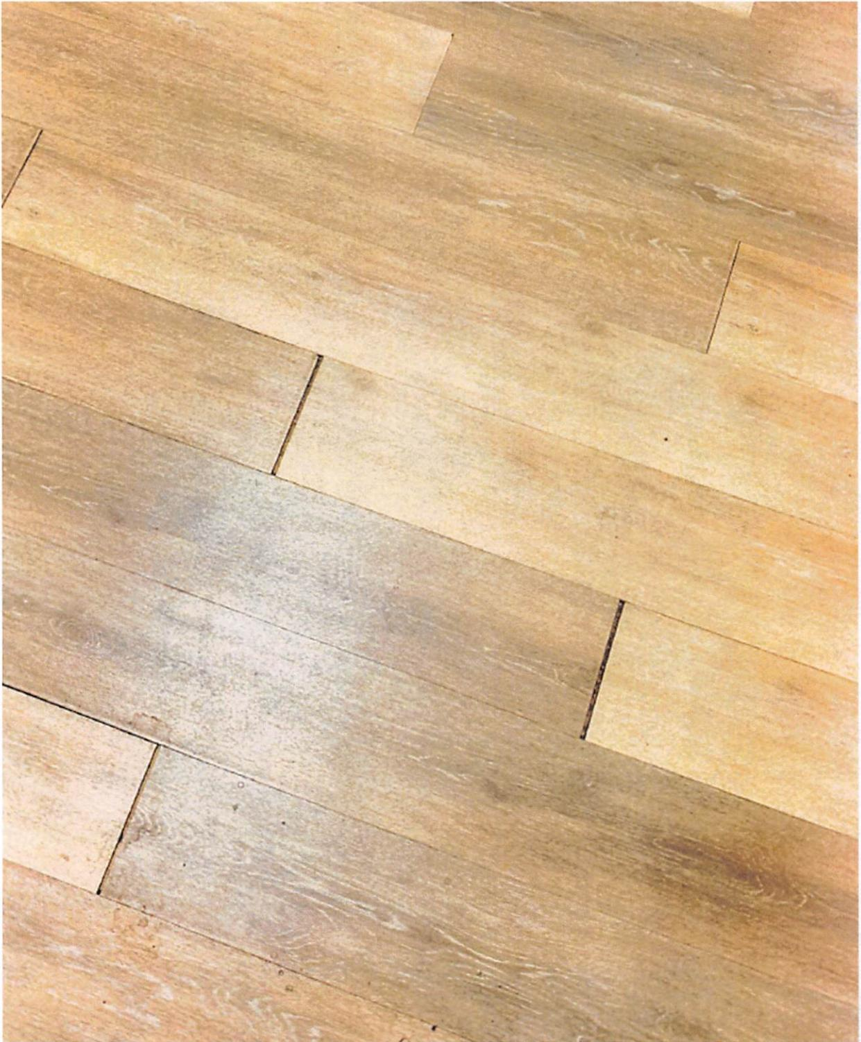
PMB FLOORING AT 3<sup>RD</sup> FLOOR ELEVATOR LANDING. THIS SECTION OF CARPET WAS REPLACED WITH GYM FLOORING DUE TO HEAVY STAINS THAT COULD NOT BE REMOVED. NOW THIS FLOOR IS BECOMING AN ISSUE AS WELL
