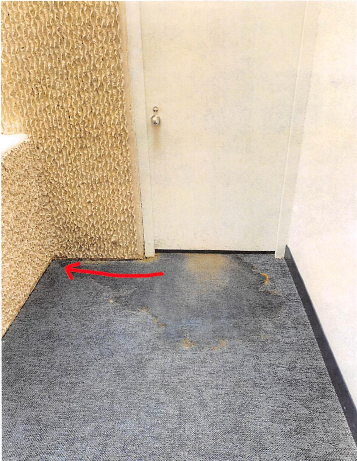
PMB ROOF AND BUILDING ENVELOPE. LEAK IS COMING FROM OVERHEAD IN THE CONCRETE THEN OUT OF THIS DOOR FRAME AND STAINING THE CARPET
