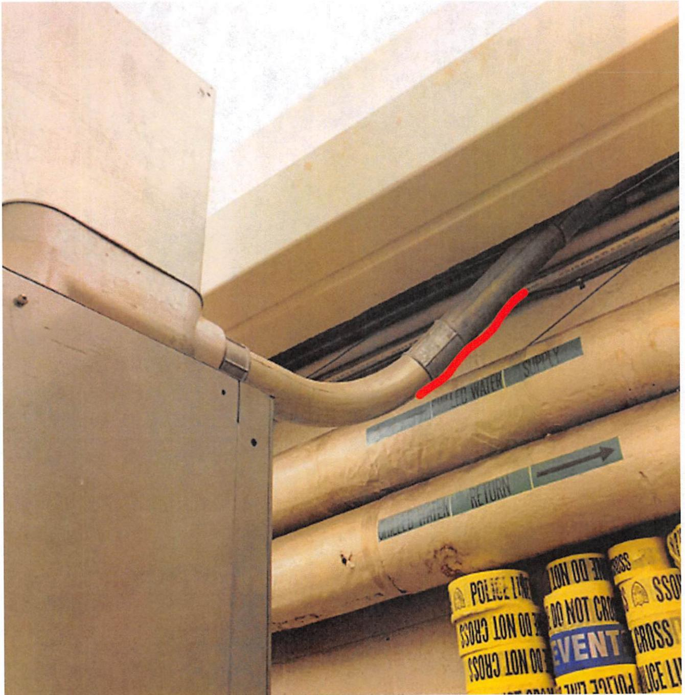
WATER FROM LEAK RUNNING DOWN CONDUITS OVER ELECTRICAL PANEL
