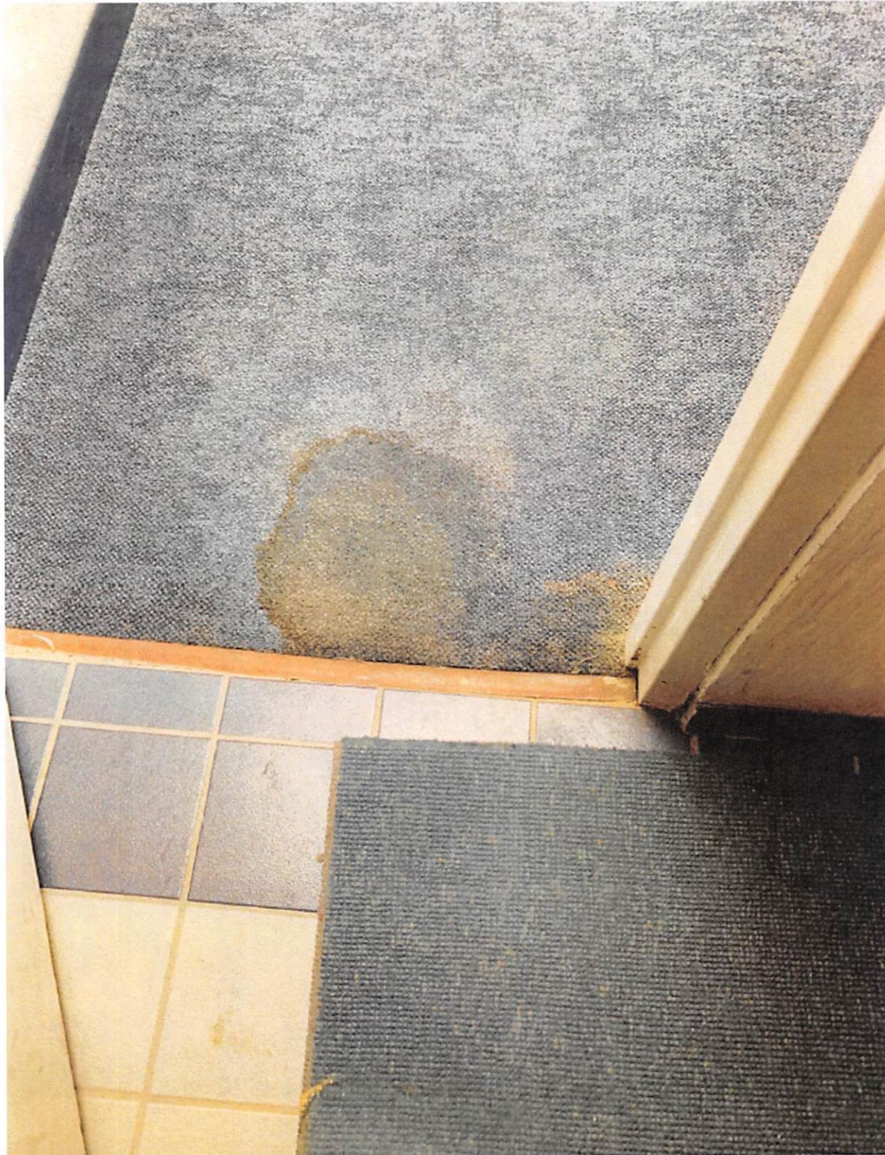
PMB ROOF AND BUILDING ENVELOPE. LEAK IS COMING FROM OVERHEAD IN THE CONCRETE
