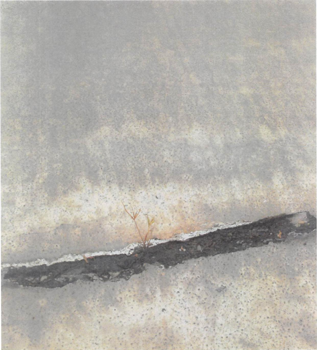
PMB HELOPAD ROOF/SURFACE IS CRACKING
