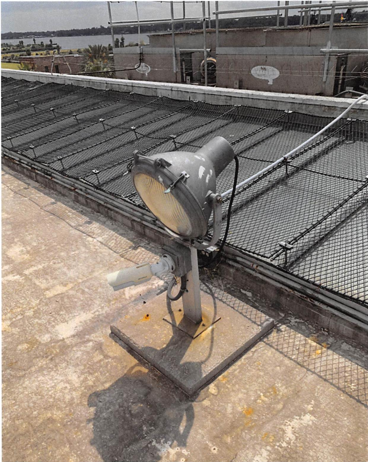
PMB HELOPAD LIGHTING SYSTEM IS AGING. SOME HAVE WATER INTRUSION IN THE FIXTURES
