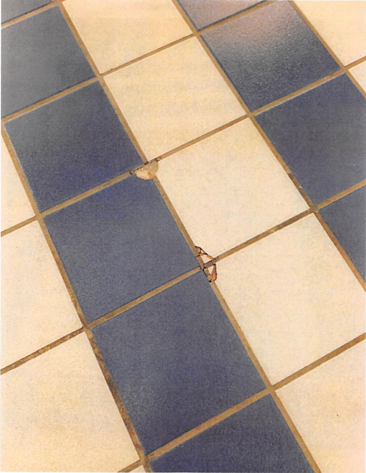
PMB TILE FLOORING IS BEYOND REPAIR. TILES ARE COMING LOOSE OR CRACKING ALMOST DAILY. THESE CAN BECOME A TRIPPING HAZARD
