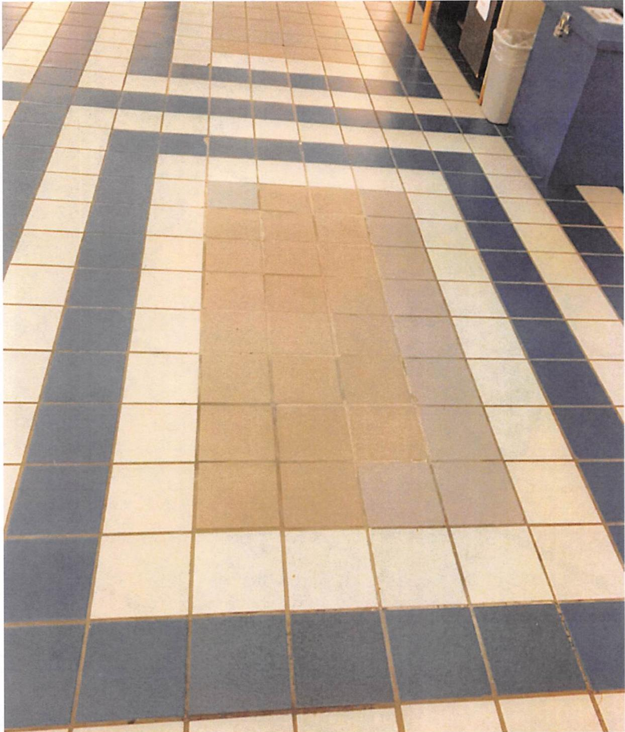
PMB TILE FLOORING IS BEYOND REPAIR. TILES ARE COMING LOOSE OR CRACKING ALMOST DAILY. THESE CAN BECOME A TRIPPING HAZARD
