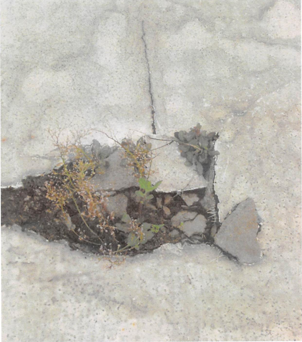
PMB HELOPAD ROOF/SURFACE IS CRACKING
