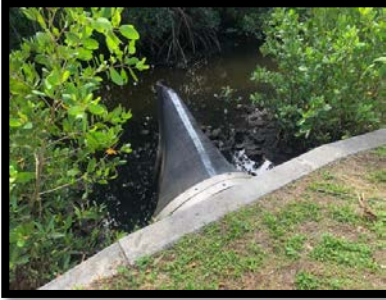
Protect Example – Backflow Valves
