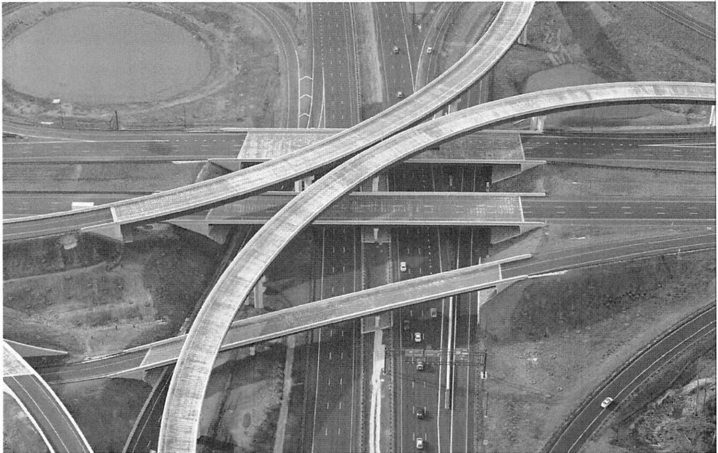
© ICC Constructors, a joint venture
